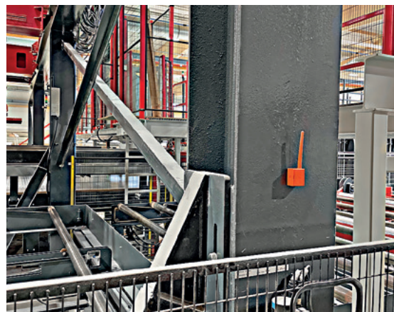
Five climate sensors ensure continuous monitoring of temperature and humidity in the production hall.
